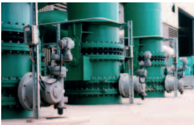
GS 500 gearboxes with primary reduction gearing and with SA multi-turn actuators in a desulphurisation unit of an Australian power plant.
